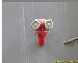
Photo of fire safety equipment Fire hydrant system.jpg
