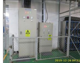
2019-12-26 09:21 Photo of fire safety equipment Electrical panel was marked with warning sign.jpg
