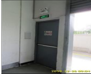
Photo of fire safety equipment Emergency exit.jpg
