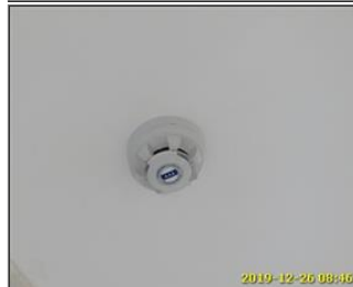
Photo of fire safety equipment Smoke detector.jpg
