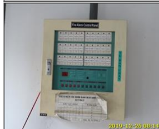
Photo of fire safety equipment Fire alarm control panel.jpg
