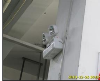
Photo of fire safety equipment Emergency light along the pathway.jpg
