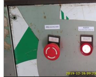
Photo of fire safety equipment Emergency stop button was labelled.jpg
