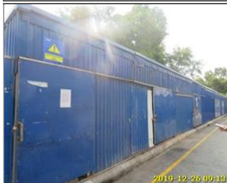
2019-12-26 09:10 Photo of the sanitary facilities Hazardous waste warehouse.jpg
