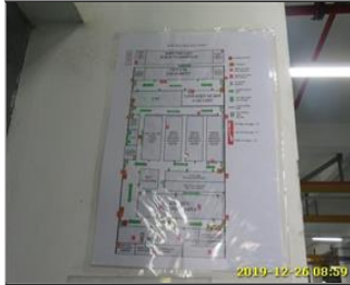
Photo of fire safety equipment Evacuation map.jpg
