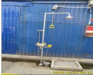
2019-12-26 09:16 Photo of chemical storage room (if applicable) Eyewash and shower station.jpg
