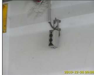
2019-12-26 09:08 Photo of fire safety equipment Beam detector.jpg
