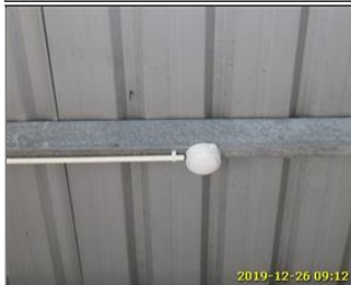
Photo of fire safety equipment Heat detector.jpg
