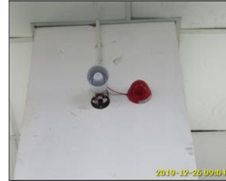
Photo of fire safety equipment Fire alarm bell and beacon flash light.jpg
