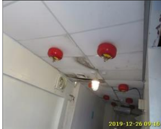
2019-12-26 09:16 Photo of fire safety equipment Automatic fire extinguisher.jpg
