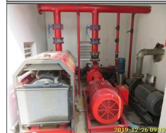
Photo of fire safety equipment Fire pump.jpg
