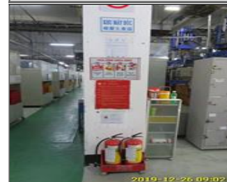
Photo of fire safety equipment Fire extinguisher.jpg
