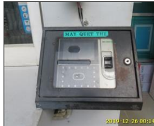
Photo of the inside of the main production hall Fingerprint machine system.jpg
